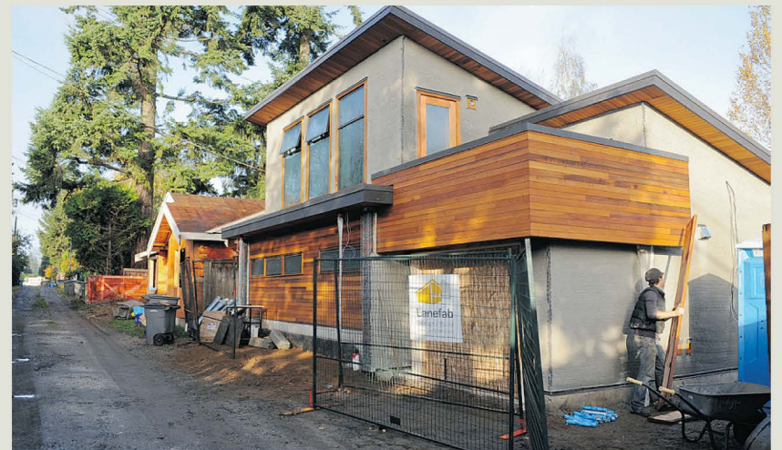
A laneway home was built in the 4600-block of West 11 Ave.
